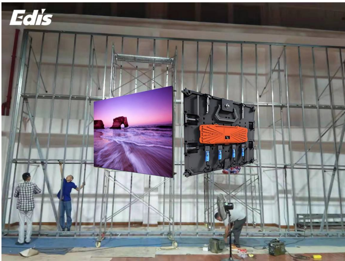
Indoor cabinets can be mounted on a steel framework as above or directly wall mounted with screws
